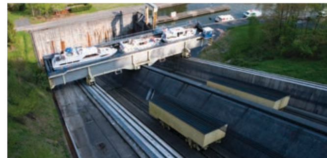
Marvel of modern engineering – the St-Louis / Arzwiller Boat Lift.
